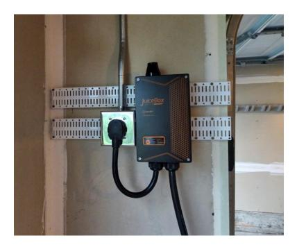
EVSE is the standard industry term for referring to a home charger for your plug-in vehicle. Pictured above is an example. It is the hardware needed to supply power from the electric outlet to the battery. Choices vary greatly, from basic & slow to providing very fast charging with remote interfaces. Prices can range from \$250 to \$1,000 units. Understanding options available will help you get the most from your purchase.
