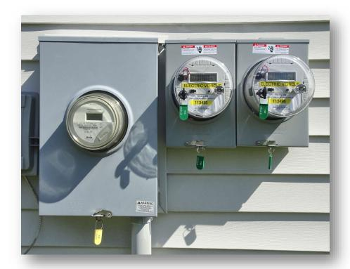
**Meters** for getting discounted charging rates from electricity providers vary. Some providers require a completely separate service, independent of your home's current setup. This can expensive to install and often includes a monthly service fee. Others only require connecting a sub-meter to the existing service.
